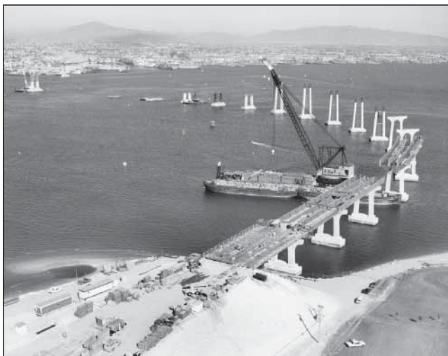
Construction of the Coronado Bridge, circa 1969
